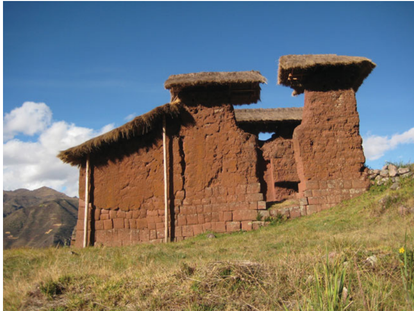
Figure 12. Huchuy Qosq'ó: Inca architecture of an extraordinary building of masonry and adobe, erected around two large natural boulders. (Photograph: J. Broda.)
